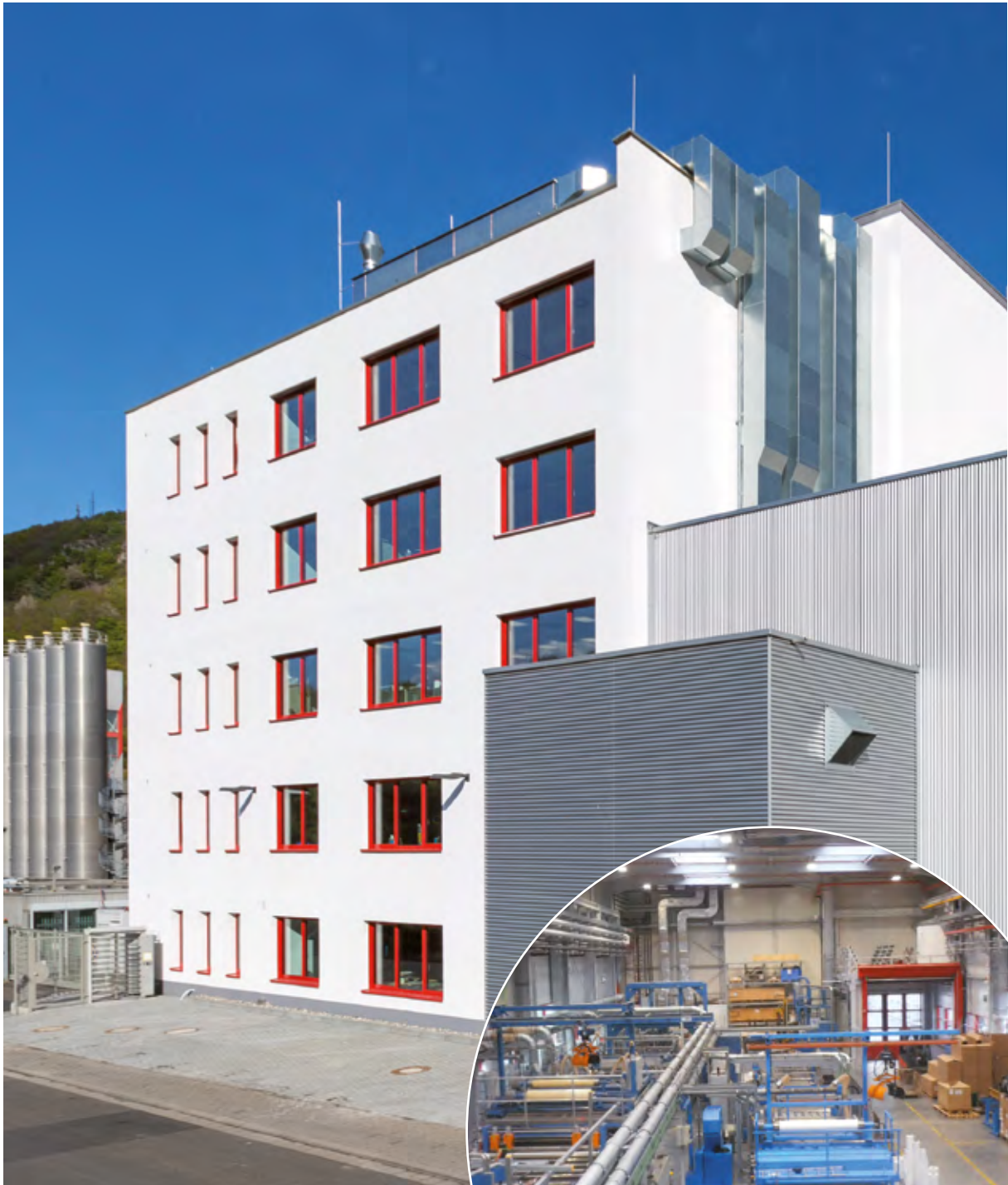
The new Technology Centre at the Kirn headquarters acts as a hub for our technical know-how, serving to accelerate our development projects.
